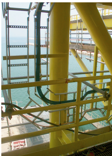
Wibe KHZP tikashylly asennettuna BP/ARCO/Technip – Al Rayyan Development, Qatar.
