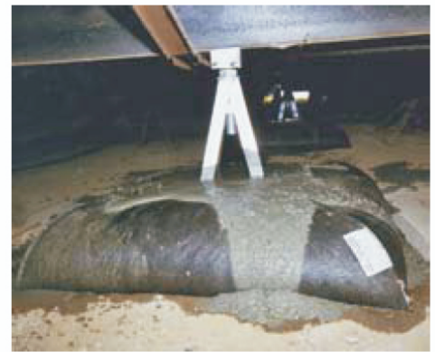
Close-up shows how concrete completely fills the geotextile bags and seeps through the bottom to form a concrete connection to the earth.
