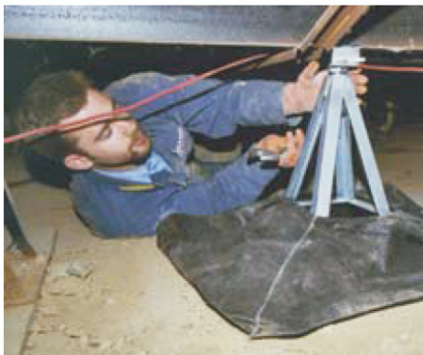
Technician completes bolting the Sure Safe steel buttress to the steel chassis beam under a HUD-Code home. Note how the base of the galvanized steel buttress is enclosed by the patented geotextile form bag.
