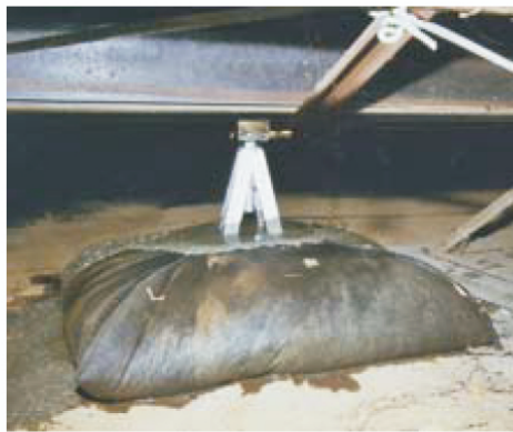
The concrete fills the bag forming a solid concrete attachment measuring approximately 6-1/4 sq. ft. At the right one of the temporary support jacks is seen which is utilized to level and hold the home firmly until the concrete hardens in the permanent buttress system members.
