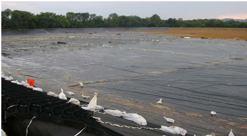
Figure 3 | Geomembrane Lined Raw Water Storage Impoundment Tennessee, USA
